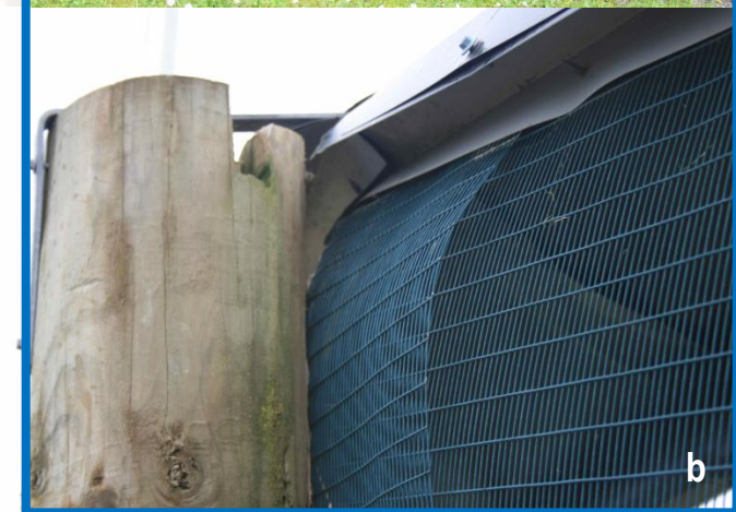
a. Jenny and Litchie off to install water collection drums. b. Damage to the fence hood.
