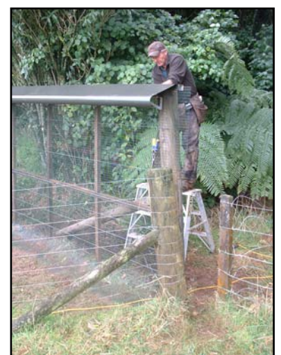
George Calvert (Xcluder) attaching the capping to the fence - Oecologico
