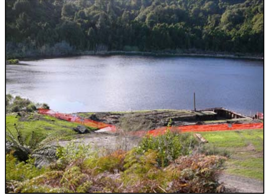
Boat ramp construction – G. Johnson
