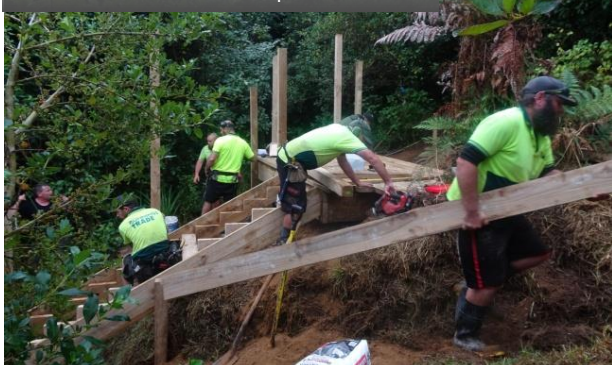
Betts & Bishop - beginning the new Bush Classroom development
